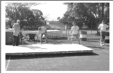
Paint Crew in Action
