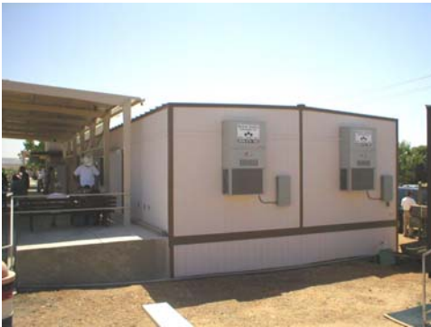
West end of new Clubhouse
