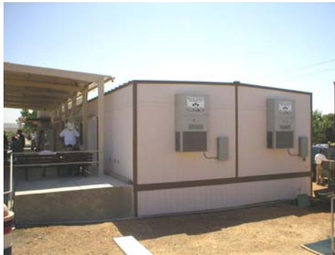
Our new Clubhouse being installed!
