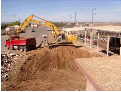
Our old Clubhouse being torn down!
